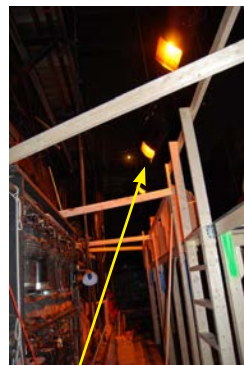
Incandescent stage lights use gel sheets attached to the casing to achieve colorization.
